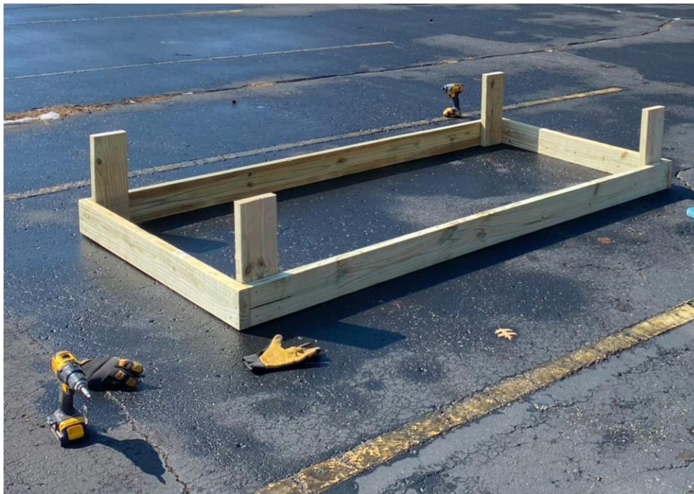
Figure 4: Raised Bed Assembly
